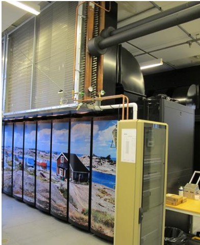
Cray XE6 "Lindgren": hot air \Rightarrow ventilator hoods \Rightarrow heat exchanger coils \Rightarrow water \Rightarrow Chemistry building
